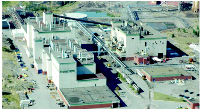
Copper Cliff Nickel Refinery, Ontario, Canada
